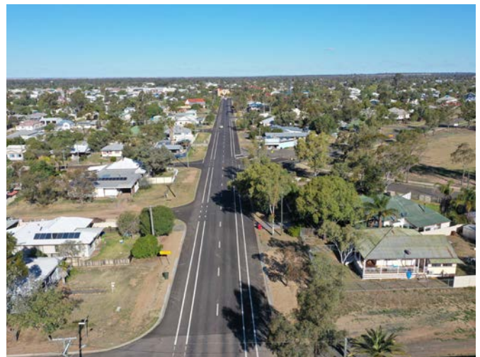
Asphalt Surfacing of Queen Street, Roma
