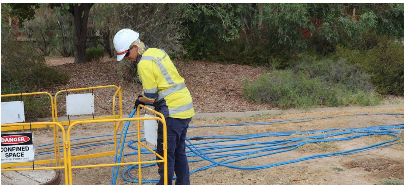
Sewer relining works in Roma
