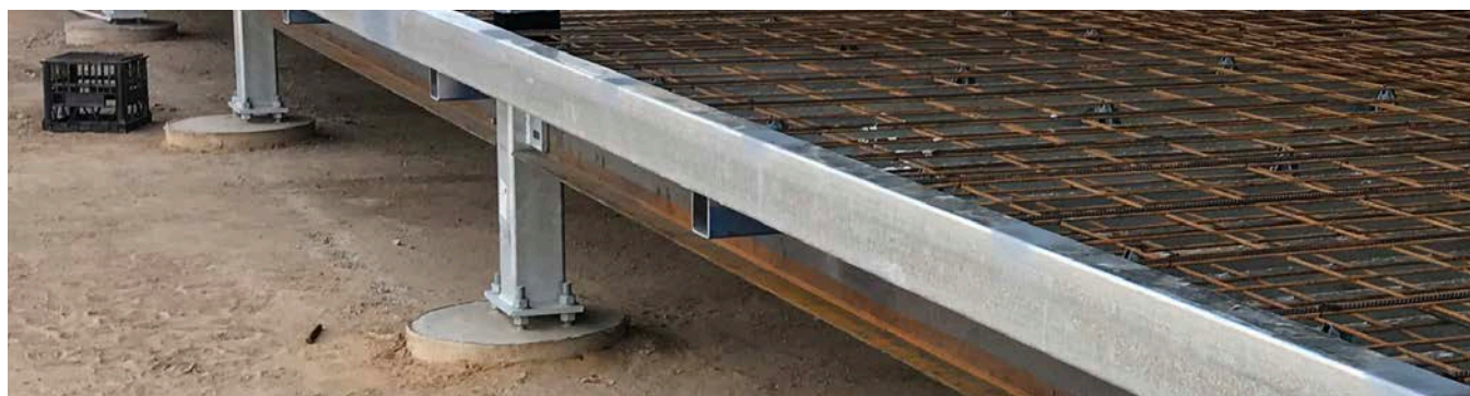
Building works in progress
