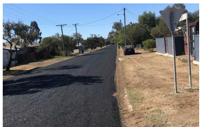
Saunders Street works completed
