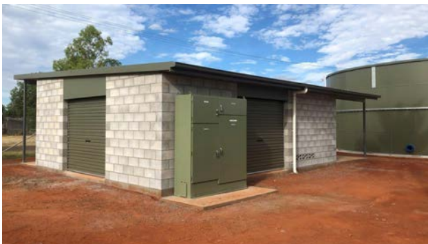
Yuleba reservoir and booster system
