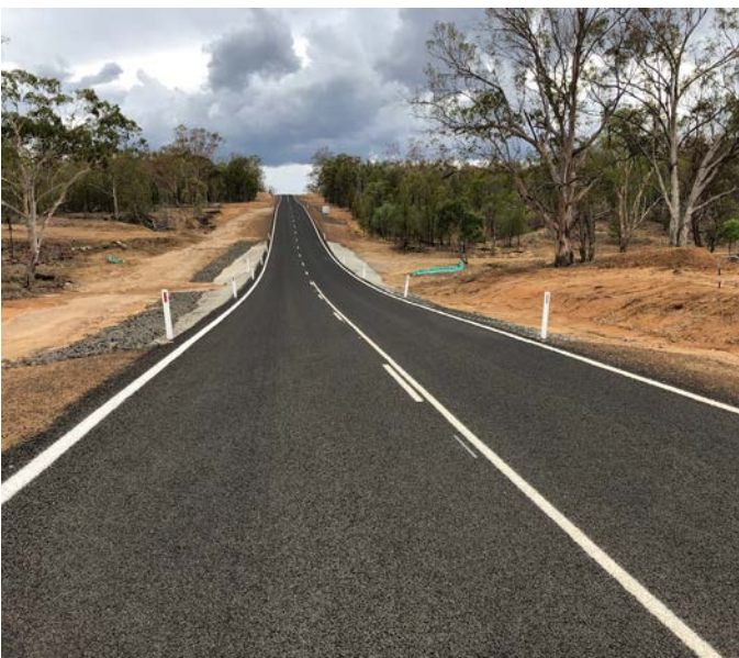
Injune Taroom Road upgrade.
