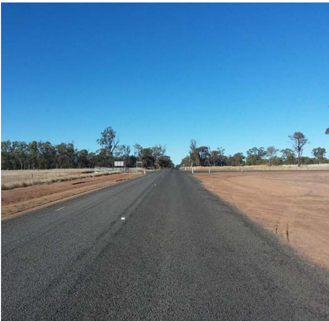
Works completed on Dargal Road, Roma
