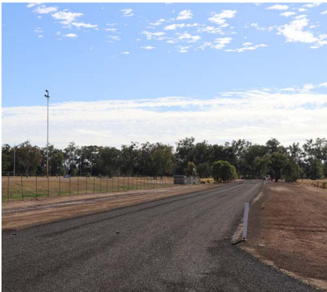
Completed works on Creek Street, Roma.
