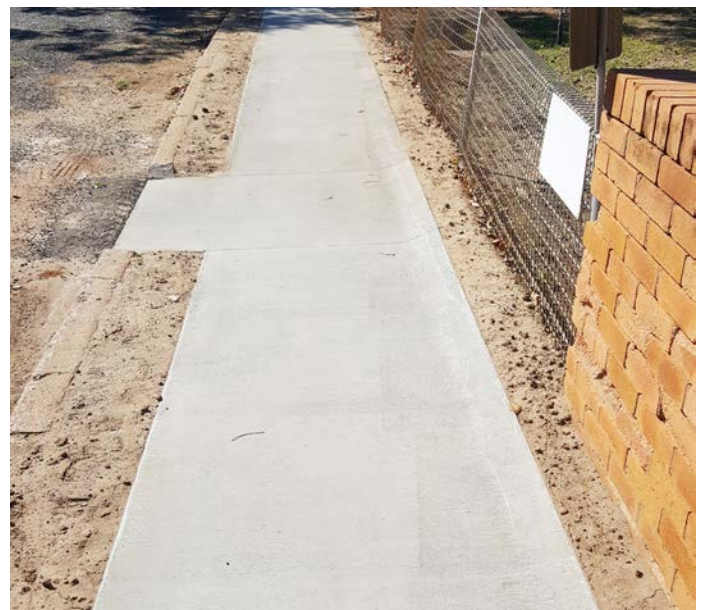
Footpath now complete in Surat
