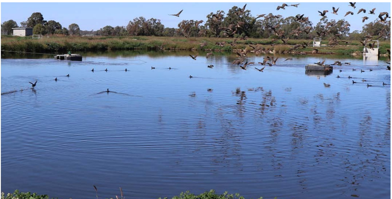
Sewage treatment, Roma - evaporative ponds
