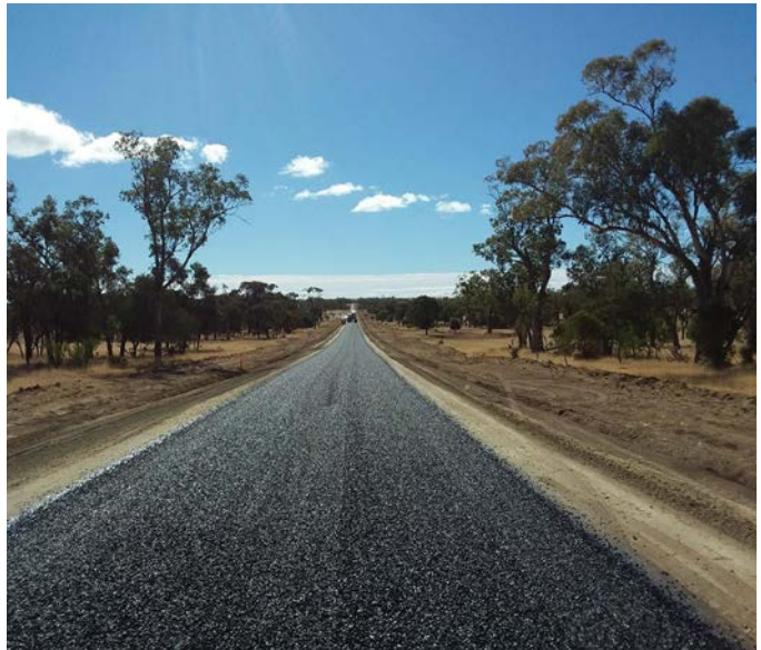
Mt Moffatt Road upgrade.
