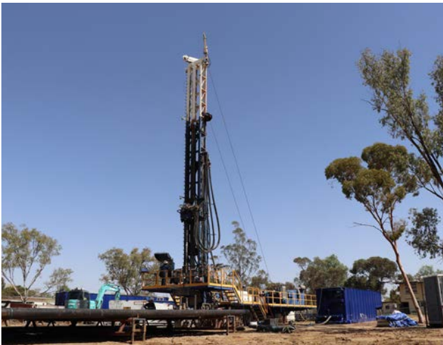
Drilling on Bore 20 in Roma
