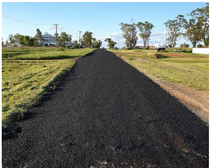
Bitumen reseal of West Street, Wallumbilla
