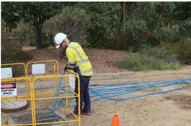
Sewer relining works in Roma.
