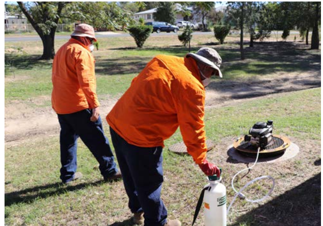
Council staff undertake sewer fogging in Roma's sewer network.
