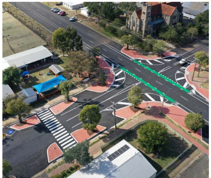
Arthur Street, Bungil Street intersection upgrade.
