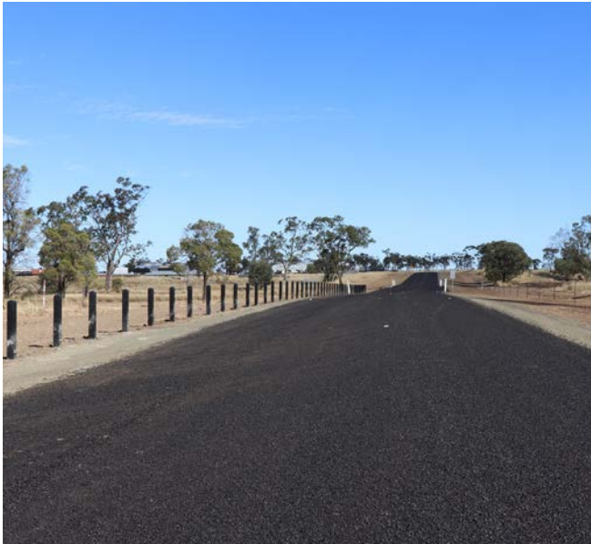
Completed works on Kimbler Road, Roma.
