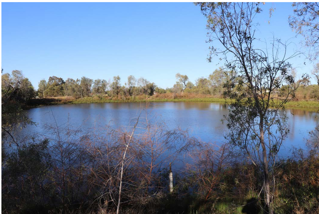
Stage 2B Flood Mitigation Site - Railway Dam
