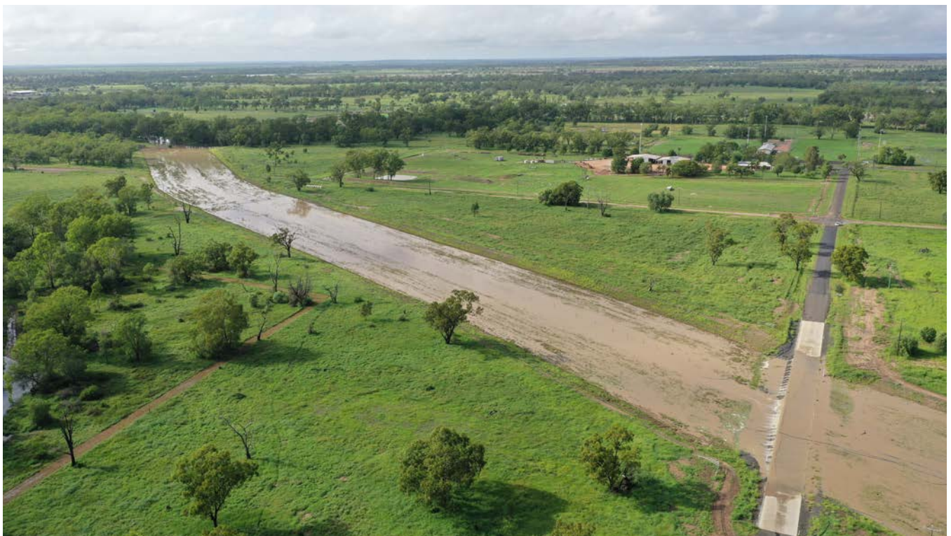
Eastern Diversion Channel - part of the Stage 2A Flood Mitigation Project, Roma.
