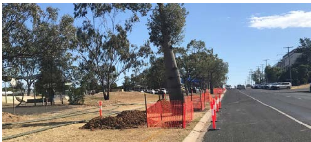
Gas Main installation works on McDowall Street.
