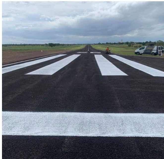
Completed reseal works on Surat Aerodrome.
