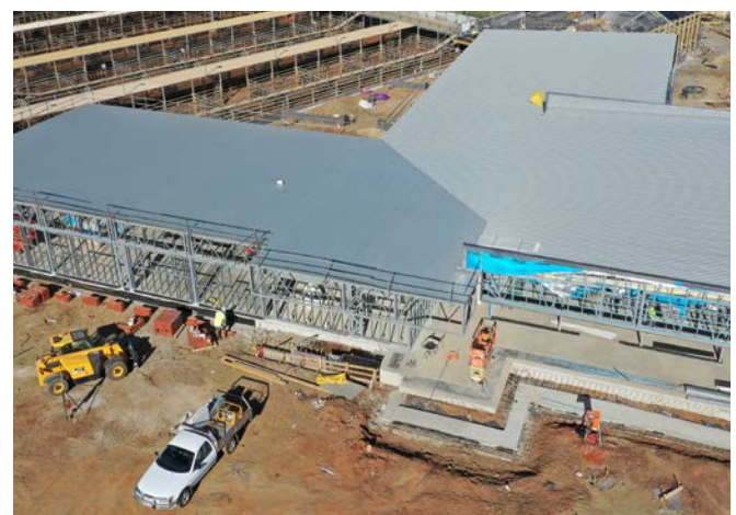
Aerial view of completion of roofing for new multi-purpose facility.
