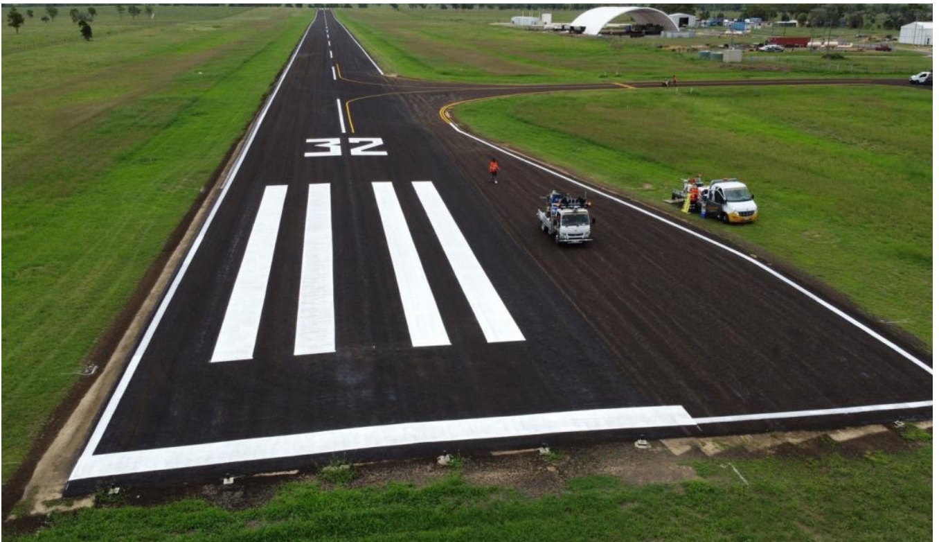
Upgraded Injune Airport Runway.
