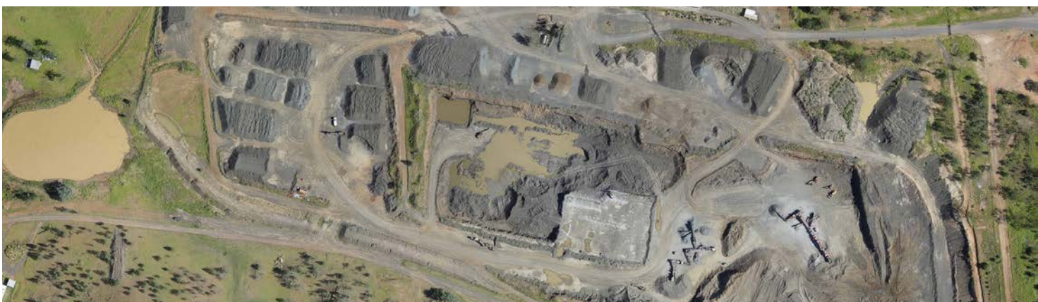
Aerial view - Roma Quarry
