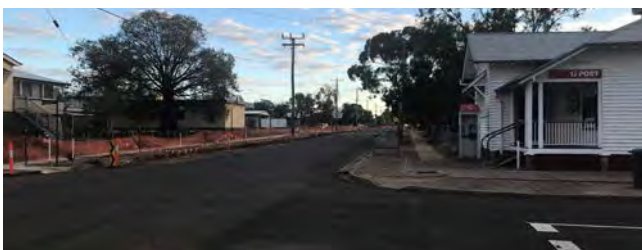
Chadford Street kerb and channel - Works in progress.
