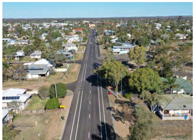
Asphalt surfacing of Queen Street, Roma.
