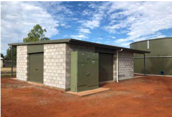
Yuleba reservoir and booster system
