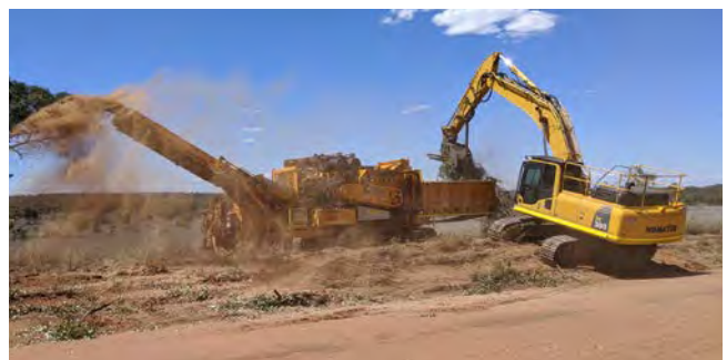
Tree clearing works on Piggery Road in Mitchell.
