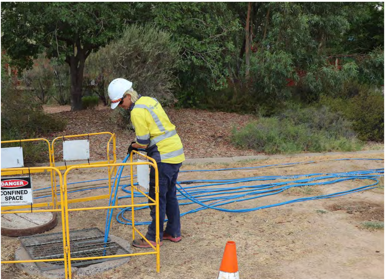
Sewer relining works in Roma.
