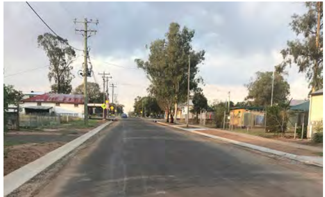
Chadford Street kerb and channel - Completed works
