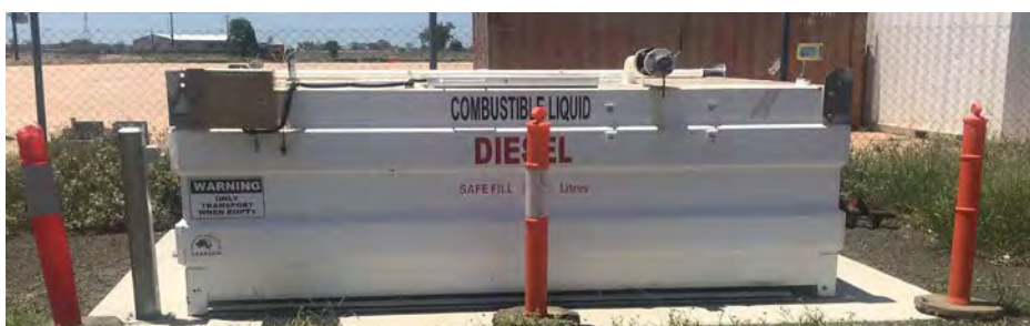
Bulk diesel tank replacement - Wallumbilla Depot (installed and commissioned).
