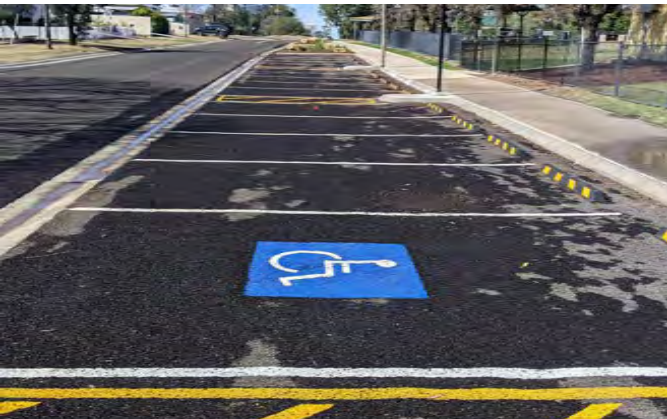
Apex Park carpark works completed.
