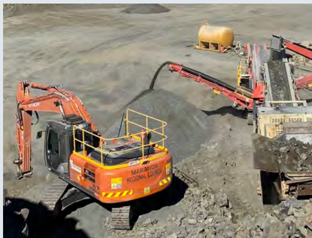
New excavator in use, Roma Quarry- Part of Council's 2020/21 Plant Investment Program.
