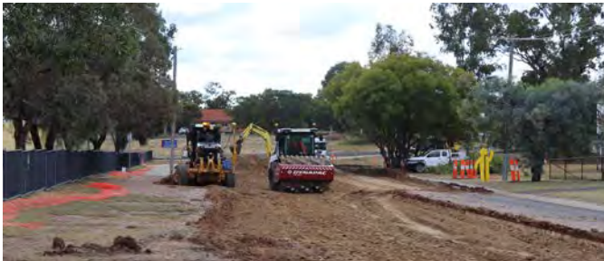
Apex Park carpark works underway.
