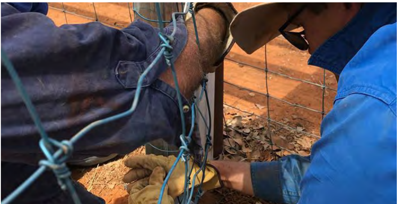
Exclusion fencing construction.
