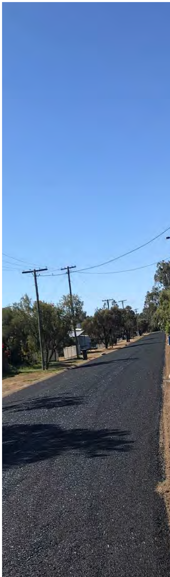
Saunders Street works completed
