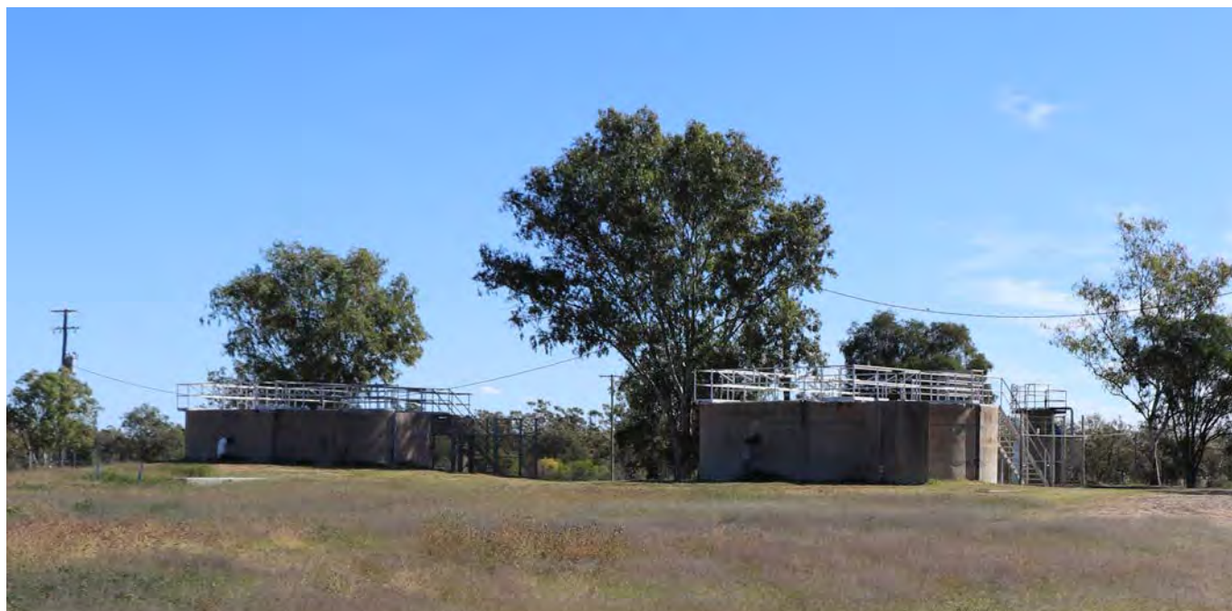
Sewage treatment, Roma - Imhoff tanks
