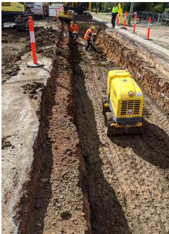
Saunders Street works in progress
