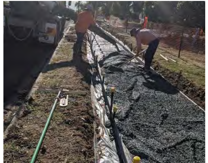
Works underway on Roma's Adungadoo Pathway
