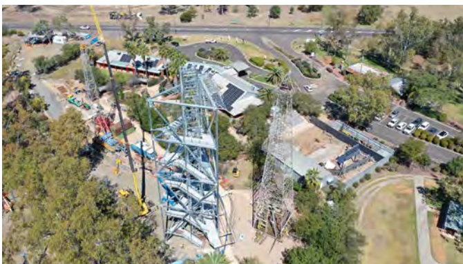
Bigger Big Rig construction
