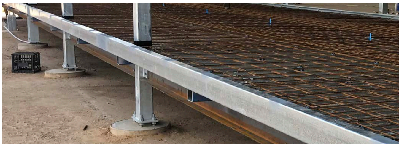
Building works in progress.
