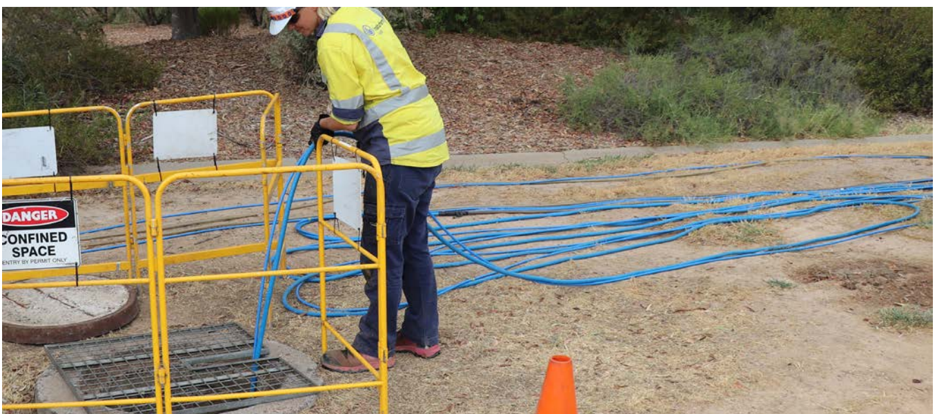
Sewer relining works in Roma
