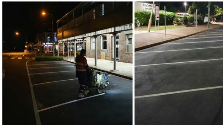
Hawthorne Street, Roma, Asphalt Overlay Project underway
