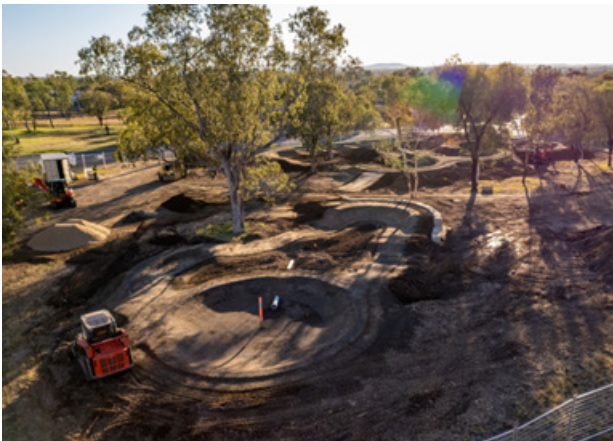
Roma Pump Track under construction
