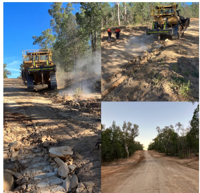
Mt Moffatt Road gravel resheeting project. This project was funded by TIDS, and saw four sections of Mt Moffatt Road upgraded.
