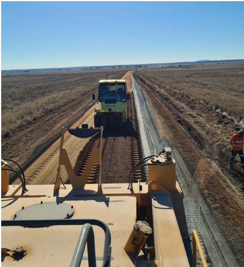
Stabiliser in action at Massey Lane
