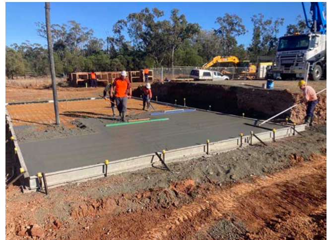
Box culvert concreting works on the Surat St George Road
