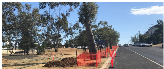
Gas Main installation works on McDowall Street.
