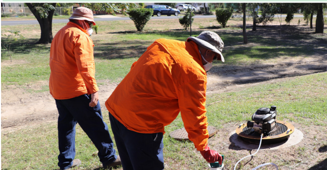
Sewer fogging in Roma.
