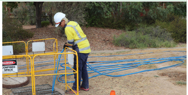
Sewer relining work in Roma.
