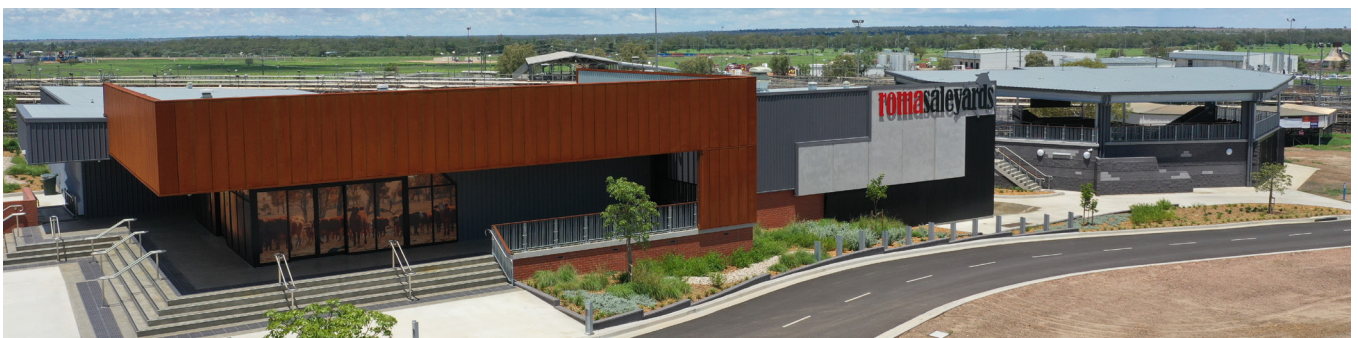
Roma Saleyards Multi-Purpose Facility.
