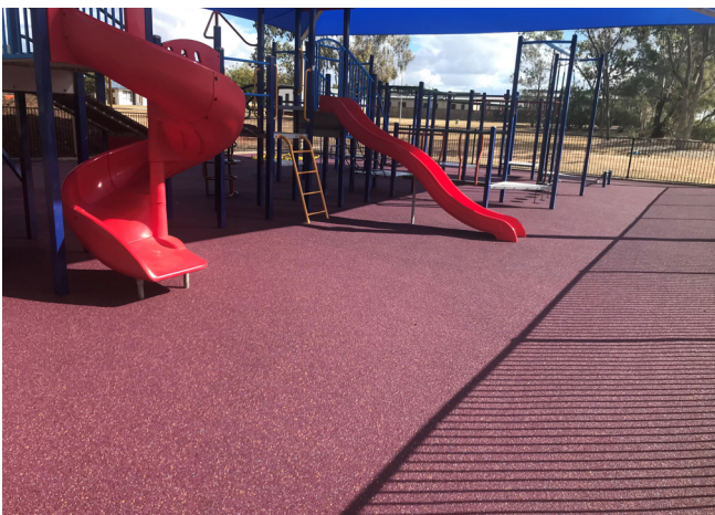
Playground (opposite hospital) upgraded with rubberised softfall.
