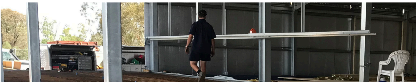
Building works in progress
