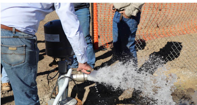
The installation of the Eumamurrin bore was completed in 2019.
