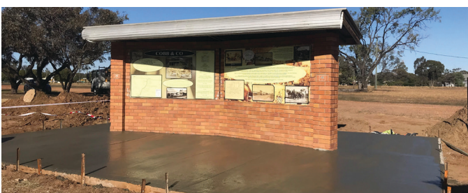
Works commence on Yuleba Cobb & Co Park redevelopment
