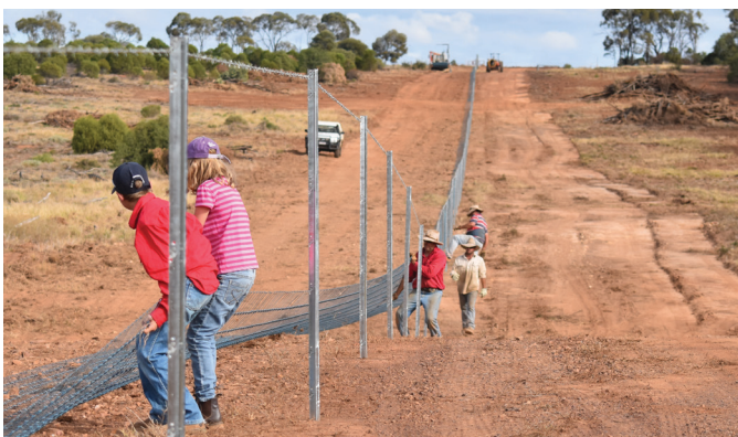
Wild dog exclusion fence project completed
