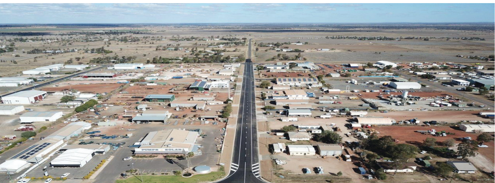
The Duke Street South Reconstruction Project, with a total cost of $2,810,692, is a joint initiative between Maranoa Regional Council, the Department of Transport and Main Roads and the Australian Government's Roads to Recovery Program which provided $281,408.
