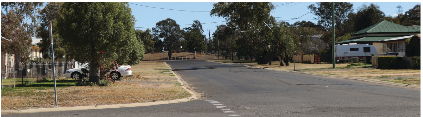
Site of gas main replacement, Roma.
