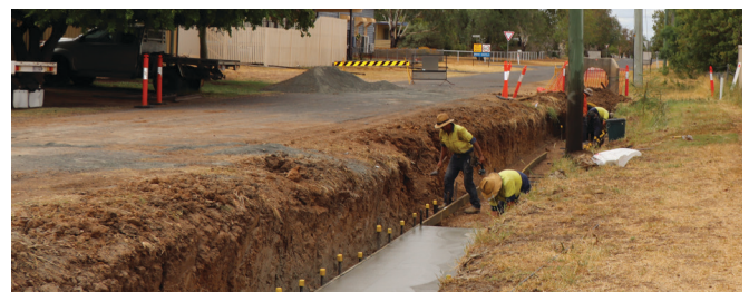
Ivy and Arthur Street intersection works improve stormwater drainage
