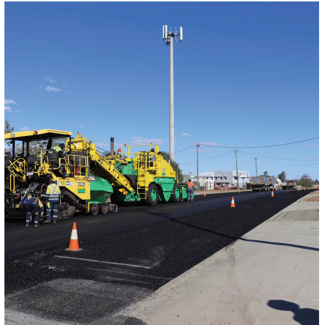
Duke Street South Reconstruction Project
