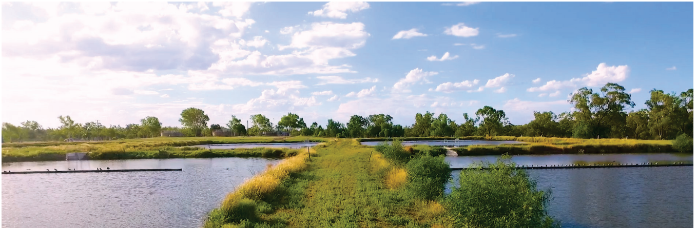
Sewage Treatment Plant, Roma.
