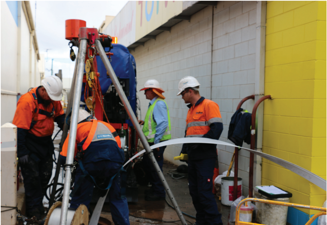
Sewer relining works.
