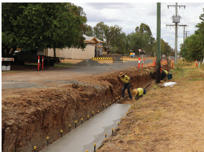
Works underway on Ivy Street.
