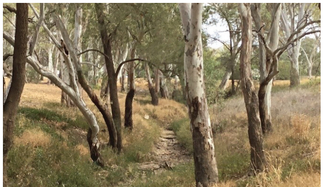
Creek precinct after clearing works (above).
