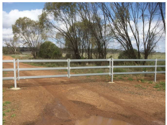
New gate and fencing at Jackson waste facility.
