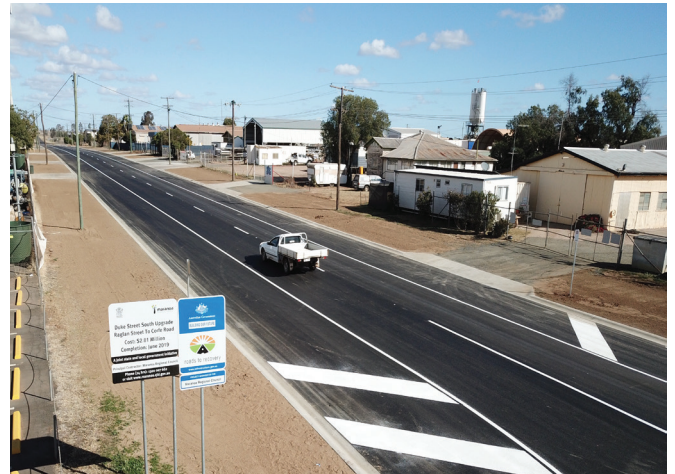
Newly upgraded Duke Street South open to traffic.
