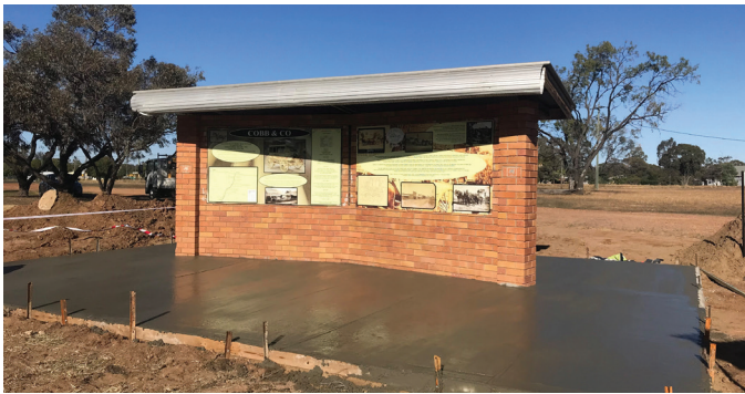
Works commencing on Yuleba Cobb & Co Park Stage 1 Redevelopment.
