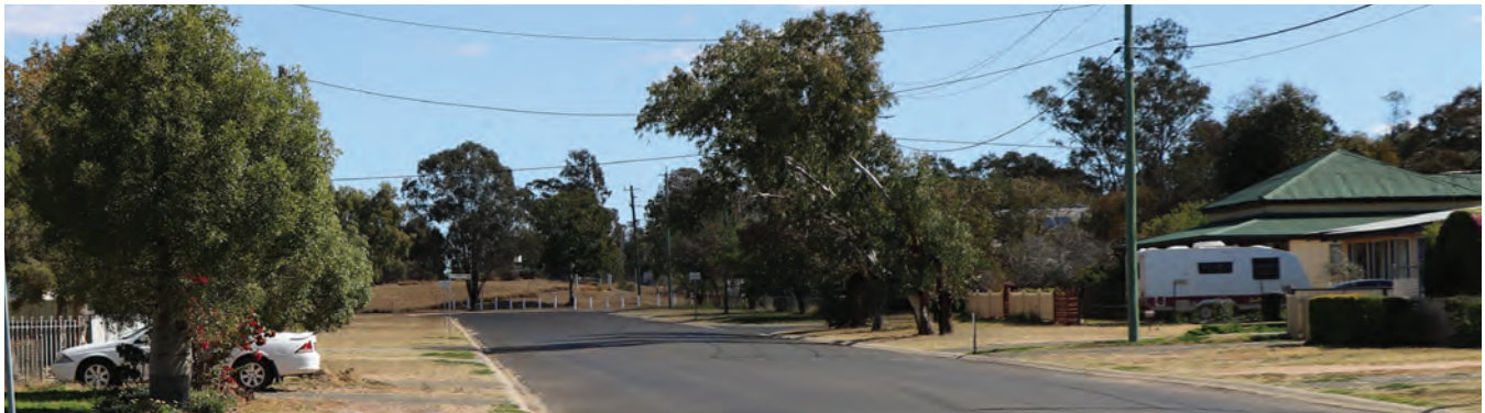
Site of gas main replacement, Roma.
