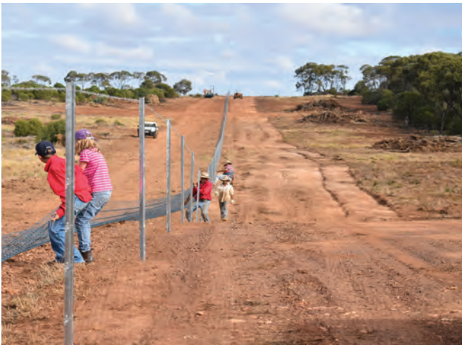
Installation of wild dog exclusion fencing.
