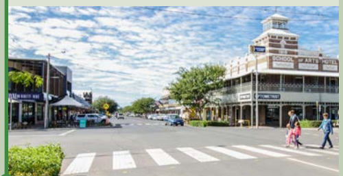
Roads and Drainage McDowall Street, Roma
