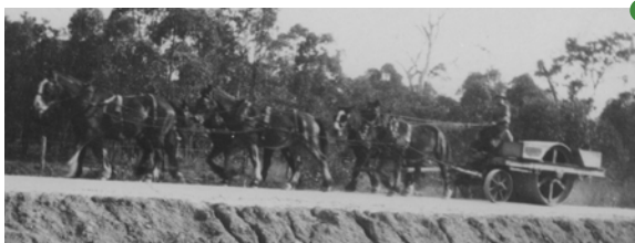
Roads and drainage Building roads, Surat - date unknown.
