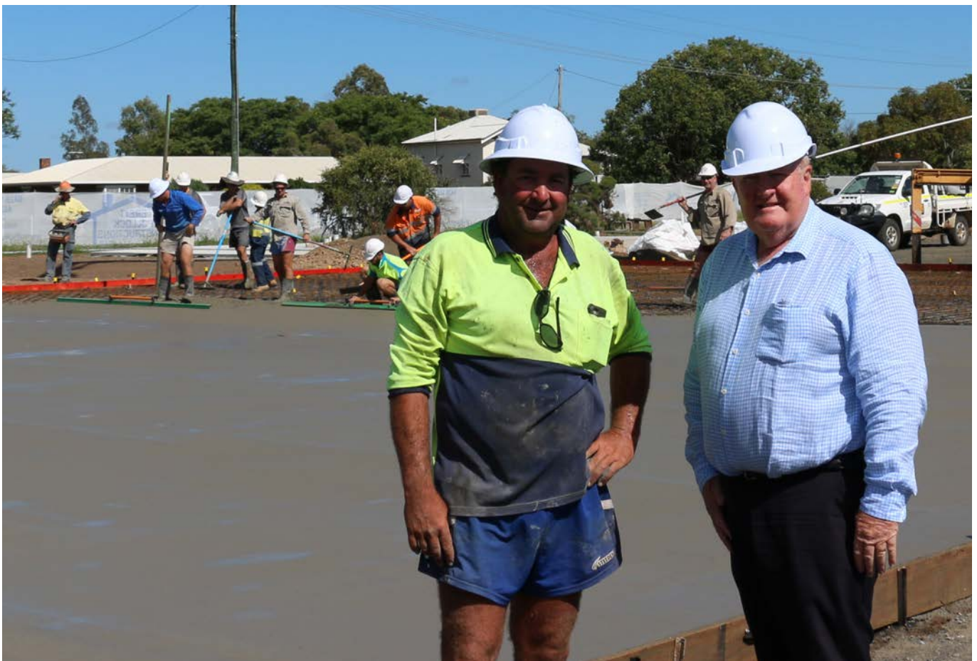
Contractor Brett Pollock and Cr Peter Flynn inspecting works at the Maranoa Netball Precinct.
