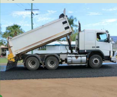
Roads and drainage Upgrading roads, Roma
