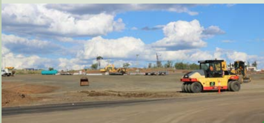
Roads and drainage Upgrading roads, Roma Saleyards
