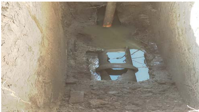
Image above: Corrosion that has occurred as a result of gases being emitted from sewage. The gas has eroded the tops of the sewer pipes. Image right: Sewer relining and CCTV works underway.
