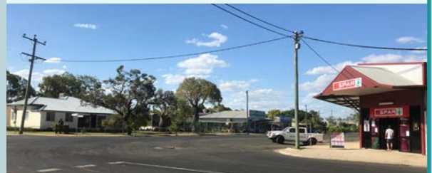
Local business Supermarket, Hutton Street, Injune
