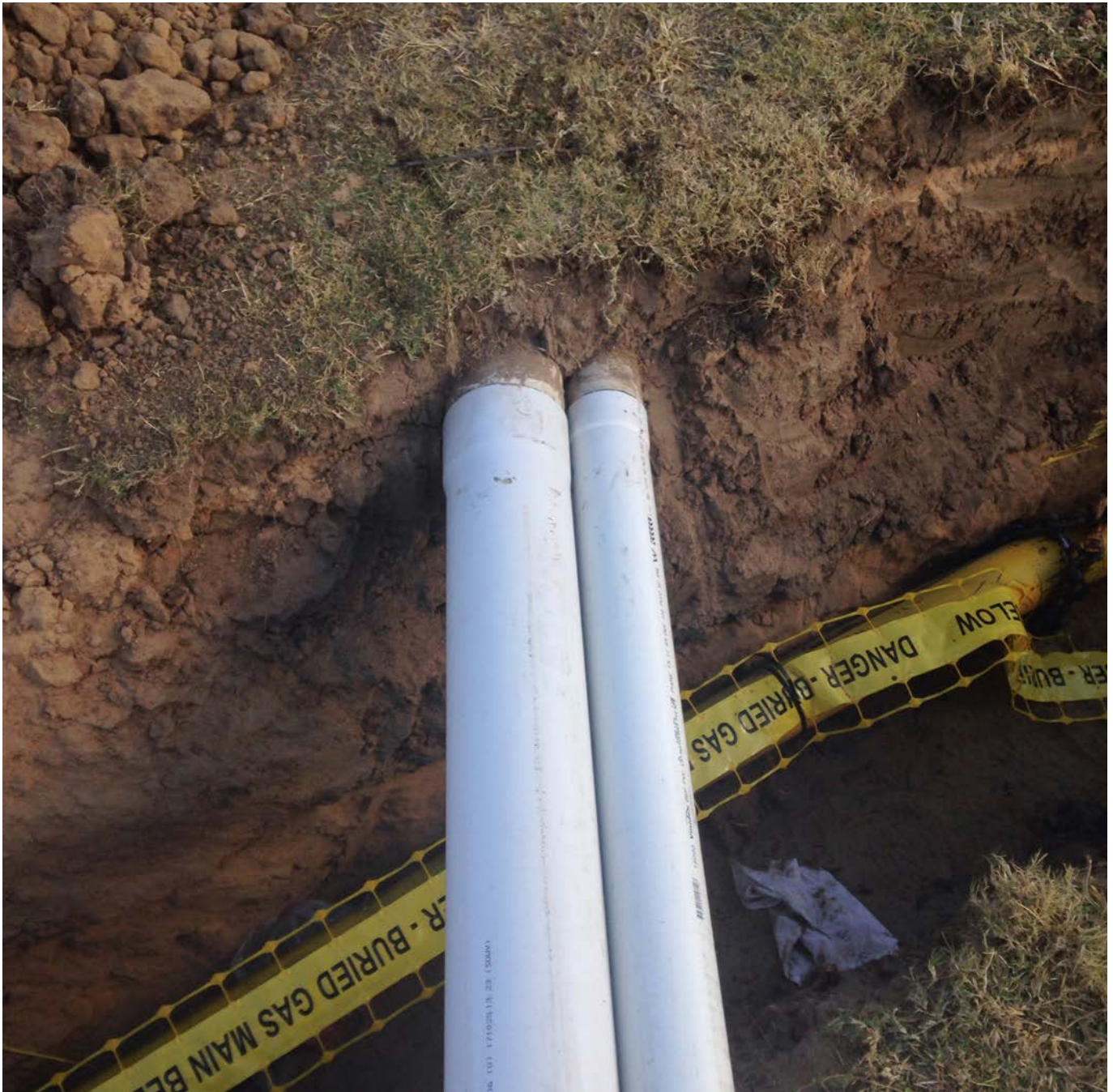
Stormwater pipes above the new gas main in Roma.
