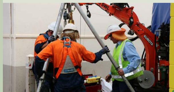
Sewerage Sewer relining project, Roma
