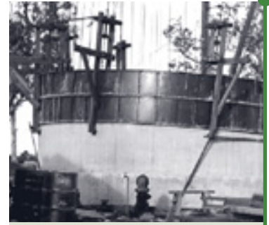
Water Water tower construction, Mitchell - 1955
