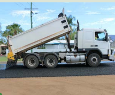
Roads and drainage Upgrading roads, Roma
