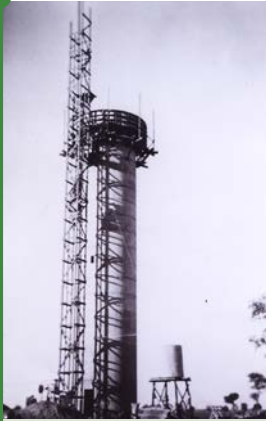
Water Water tower construction, Surat - 1951
