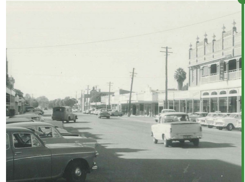
Roads and Drainage McDowall Street, Roma - date unknown.
