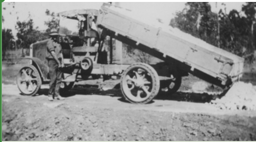
Roads and drainage Building roads, Surat - date unknown.
