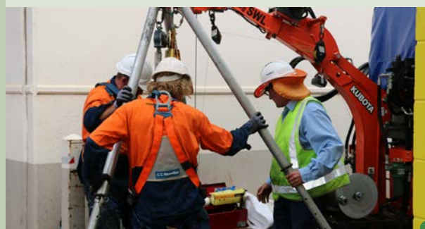
Sewerage Sewer relining project, Roma
