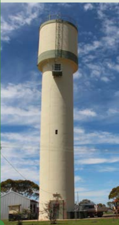
Water Water tower, Surat
