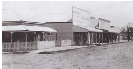
Roads and drainage Stephenson Street, Yuleba - Looking west - date unknown
