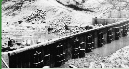
Water Construction of the weir, Surat - 1951
