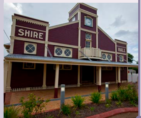
Facilities Shire Hall, Surat
